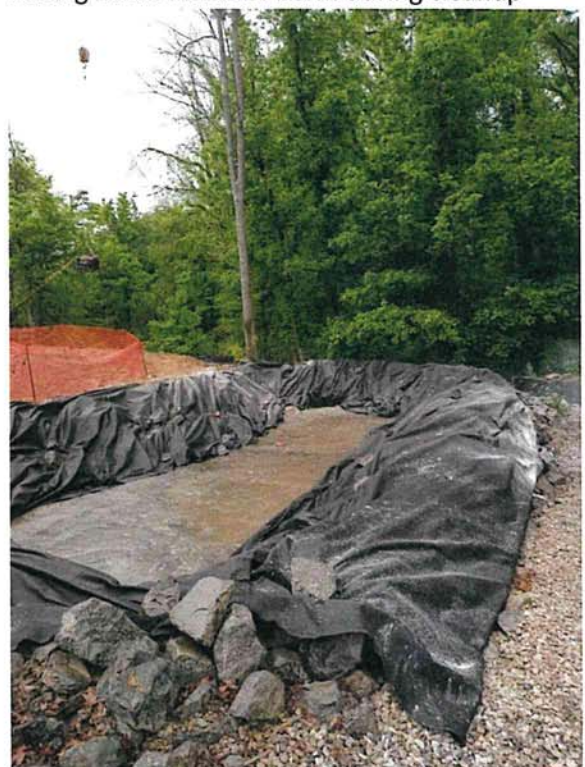
Inside berm after cleanup. The berm has been enlarged by 50%.
