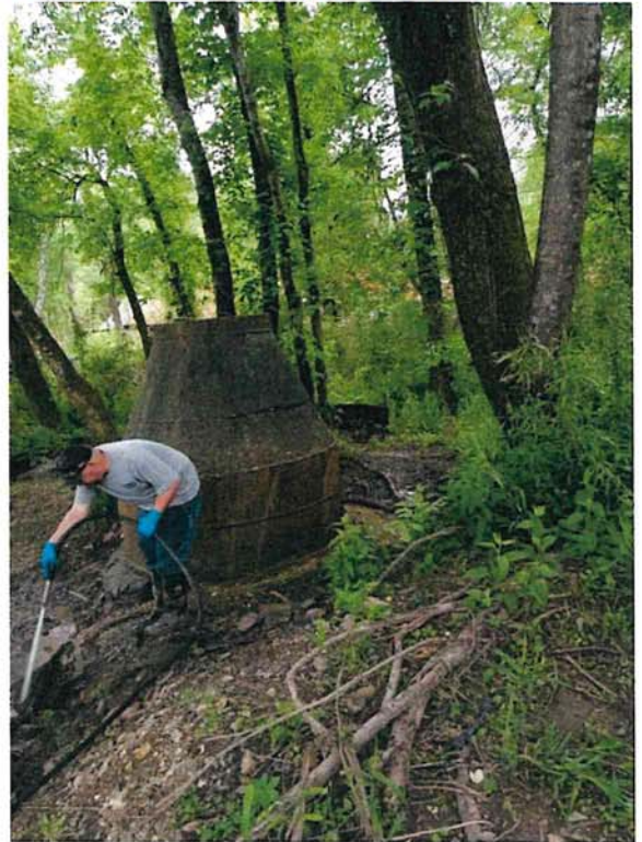
MH 1748 during cleanup
