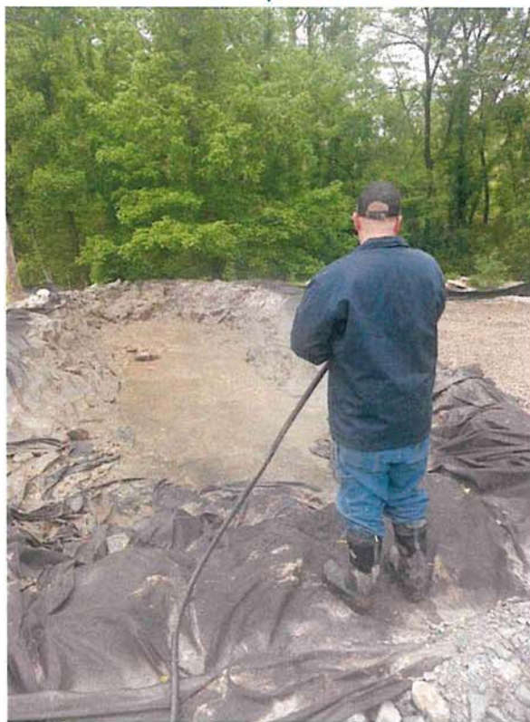
Hosing down inside of berm during cleanup
