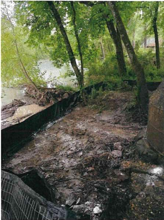
MH 1748 after cleanup with lime and new silt fencing
