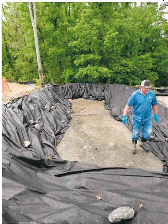
Installing new filter fabric
